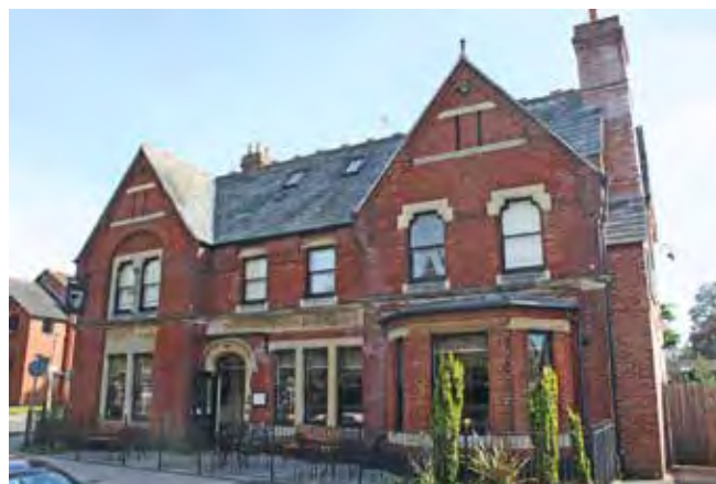
The Goods Yard public house (ex-Station Hotel)
