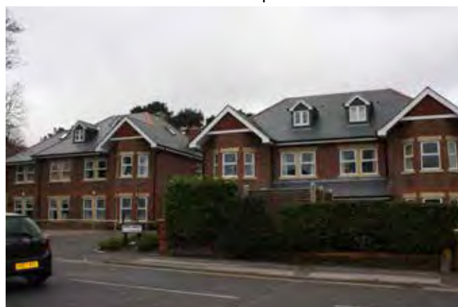
Recently built flats in York Road
