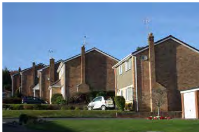
Low density housing in West Way
