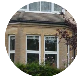
Sandstone lintels & quoins
