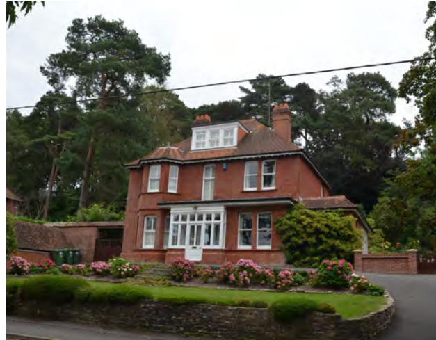
Figure 19: – A 2.5 storey house standing in extensive grounds.
